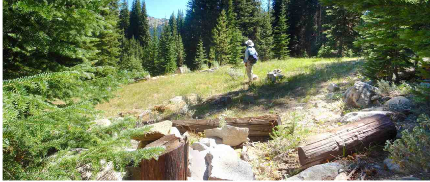
Remnants of an early-1900s power line from Fremont Powerhouse to Cable Cove can still be found here.
