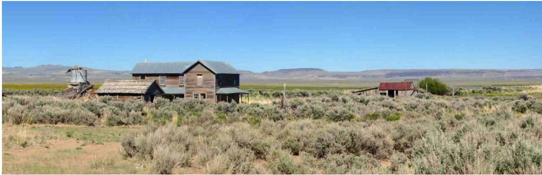
The old Shirk Ranch, bordering a series of sink lakes and wet grasslands, was abandoned in the 1940s.
